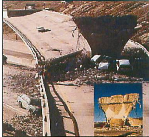
Second of 2 collapsed connector structures at I-5-SR 14 interchange.
